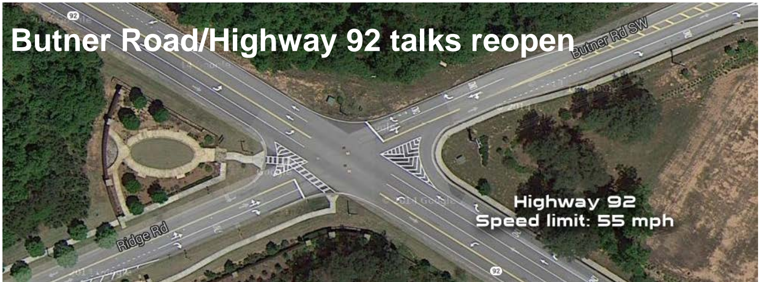
State Highway 92 at the intersection of Ridge Road and Butner Road.
